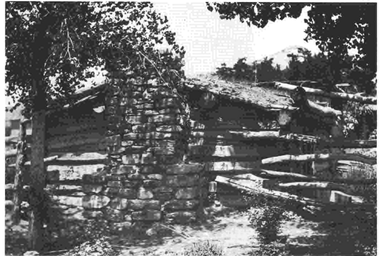
Early home in Bluff City, Utah. Constructed of crooked cottonwood logs, with a stone fireplace chimney. Gift of Neil M. Judd, courtesy Utah Historical Society.
