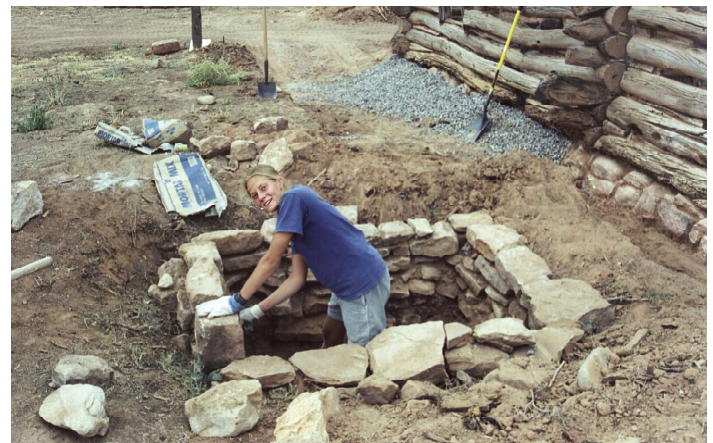
The well was partially restored using its original stones. For safety reasons, the well was only excavated down about 3 feet. Pioneer journal entries indicate that they obtained good water at 16 feet.
