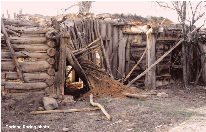
East breezeway entrance after the roof collapsed, May 1998
