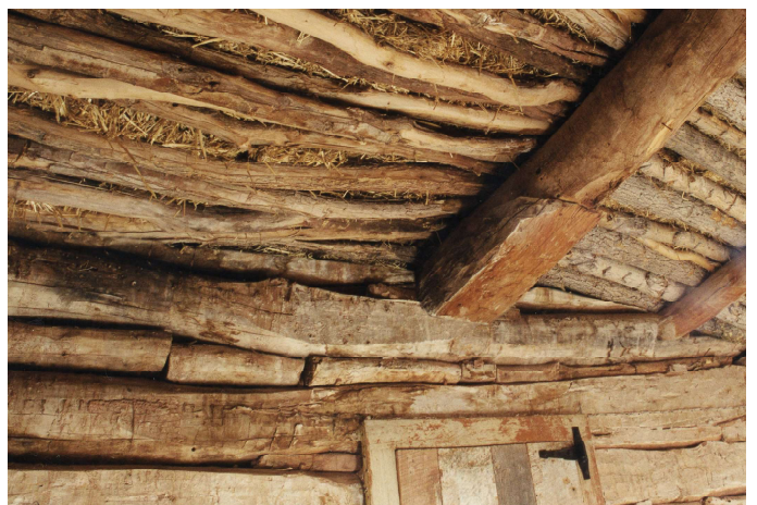
The breezeway ceiling after the center beam had been fixed and new roof logs were in place
