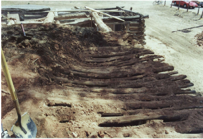
The original sod roof on the northeast cabin room was still mainly intact, but due to its condition, it was completely removed.
