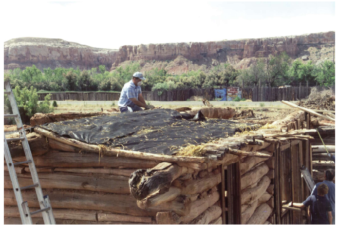
Covering new roof logs with straw and a rubber membrane
