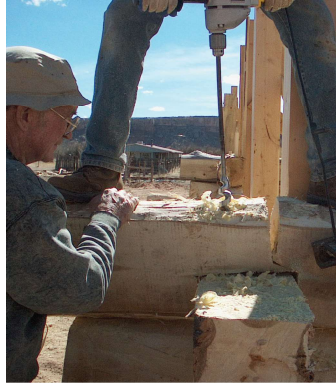
Ray Wrigget and Joe Hurst's crew securing logs with dowels (wood stakes) as the pioneers did
