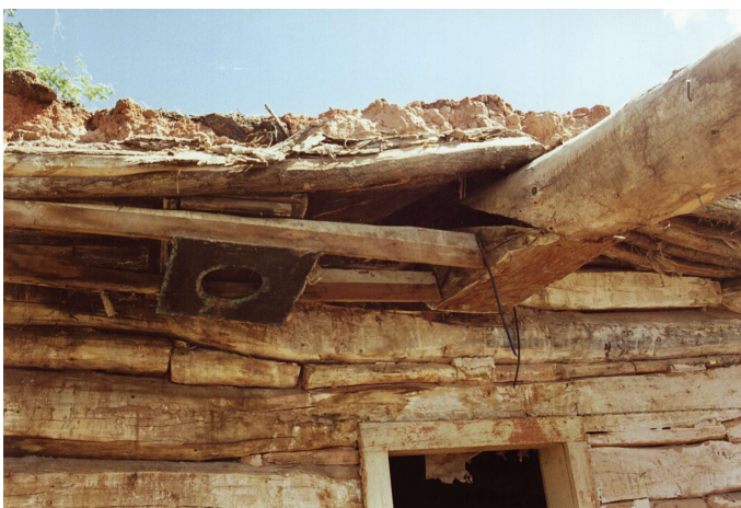
The remnants of the breezeway ceiling/roof and it's drooping center beam prior to its renovation Note the opening for a stove pipe to the left of the door opening.
