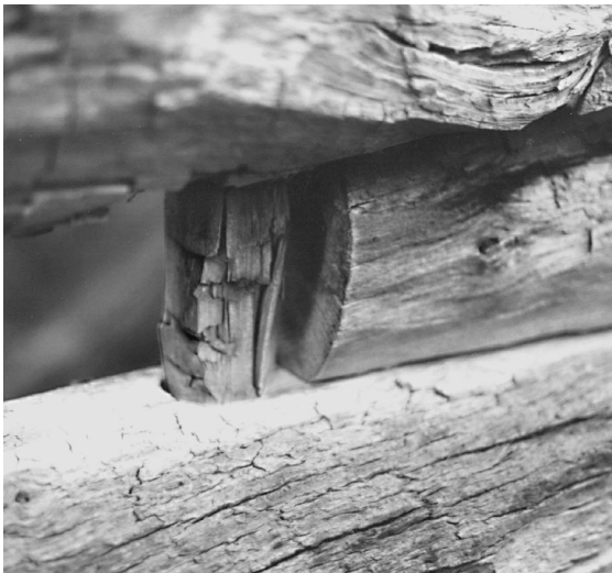
Examples of the tightly fitting pegs which added to the strength and stability of the walls.
