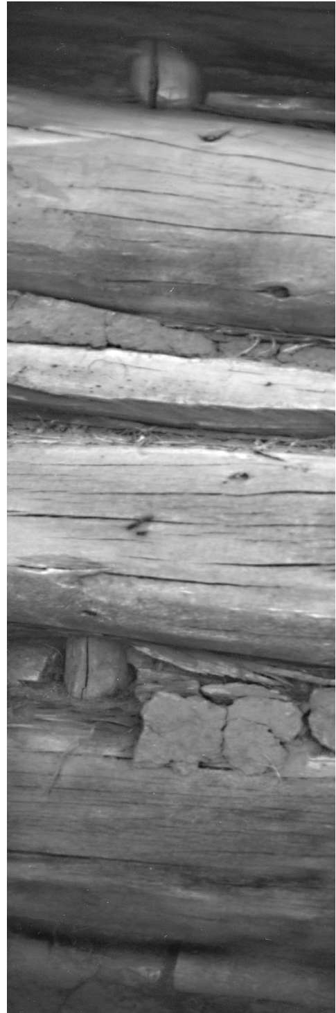
Examples of the tightly fitting pegs which added to the strength and stability of the walls.
